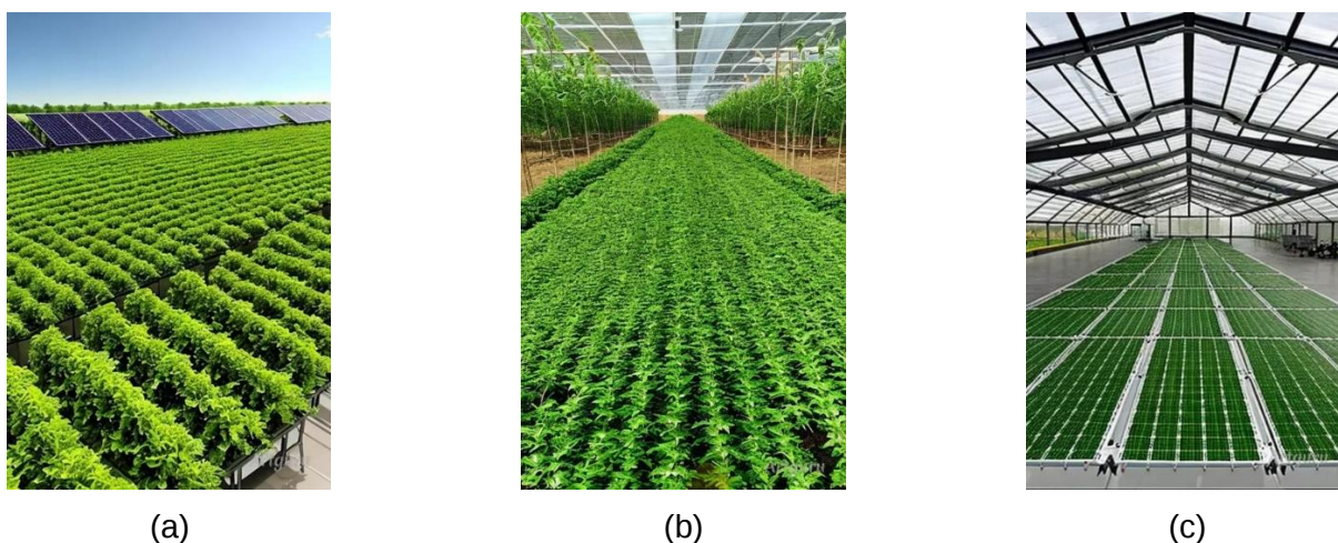
Figure 2. Assembly configuration of photovoltaic module arrays for consortium production of cultivation and photovoltaic energy by the Agri-PV system, where (a) Arrays composed of photovoltaic modules interspersed between the cultivation rows; (b) Photovoltaic modules above plantations mounted on stilts; and (c) Photovoltaic modules replacing the protective covering of greenhouses or greenhouses.
