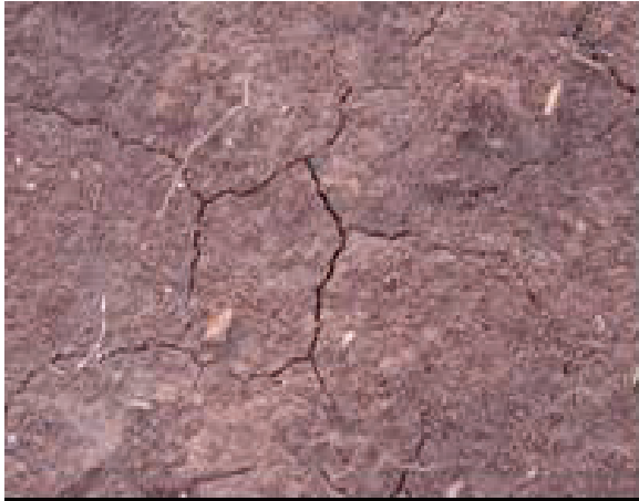
Figure 4. Fissures on the surface of NVef.
