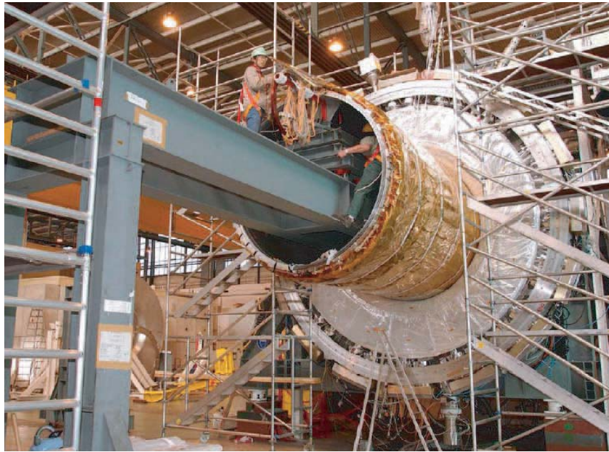
FIG. 3: LAr barrel calorimeter fully assembled. The central solenoid is being inserted into the common cryostat. In July 2004 this system has been cooled down and the solenoid was energized to its full current, including an 8% safety margin.
