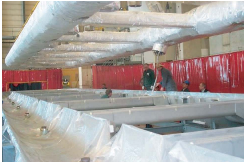
FIG. 2: Insertion of the second BT coil in its cryostat. The coil cold mass and thermal shielding are inside the multilayered insulation system wrapped around them.
