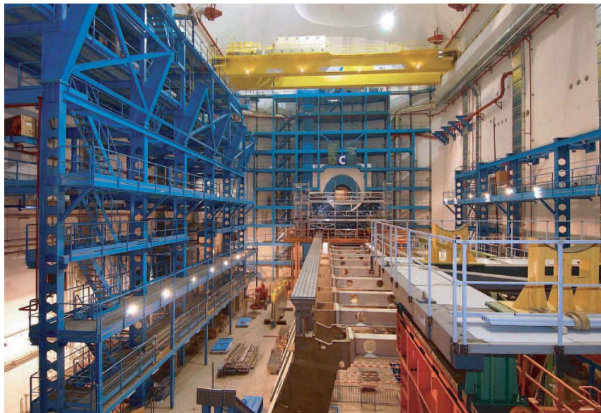
FIG. 5: ATLAS underground experimental cavern, status May 2004. Visible is the half cylinder of the barrel Tile Calorimeter, which has been assembled underground since March 2004.
