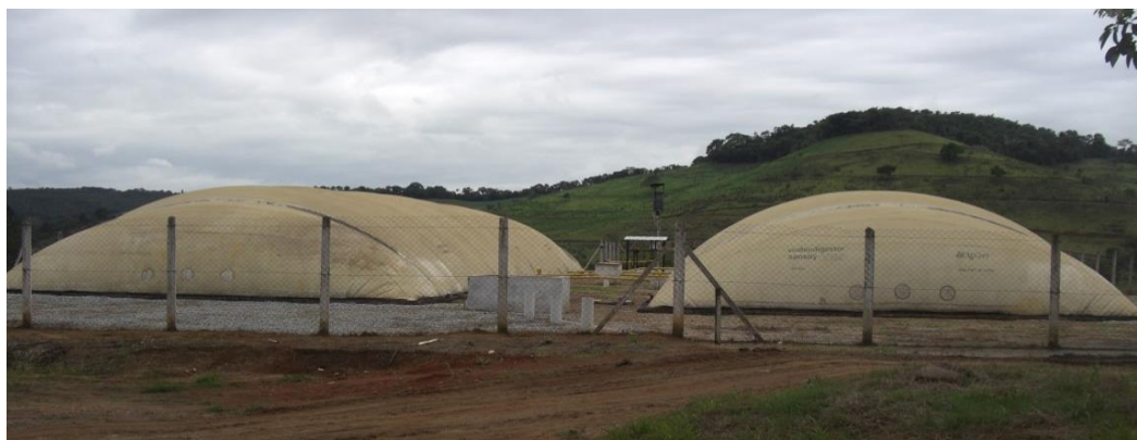
FIGURE 1. External view of the two digesters installed in farm "A".
