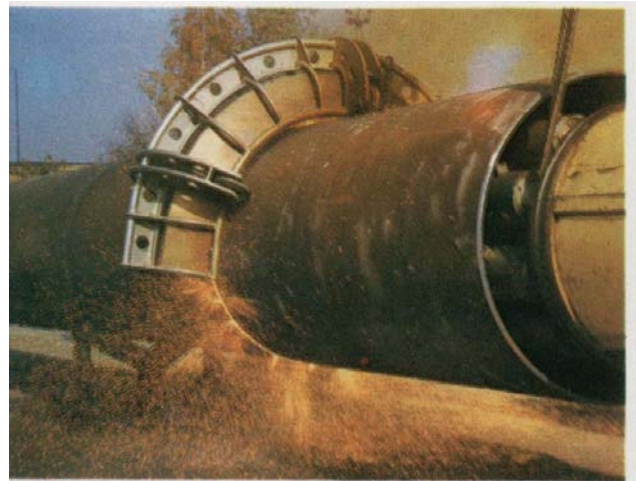
Figure 11. Flash-butt welding operation.
