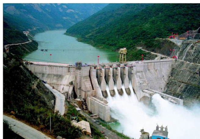
Figure 5. Dachaoshan spillway. Source: MD&A (2018).
