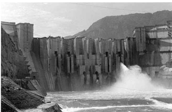
Figure 1. Slit Bucket at Geheyan Dam in China. Source: China Gezhouba Group International Engineering Co. Ltd (2010).
