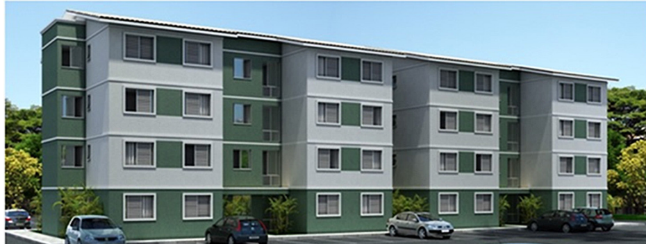
Figure 4 - Pilot building with concrete walls.
