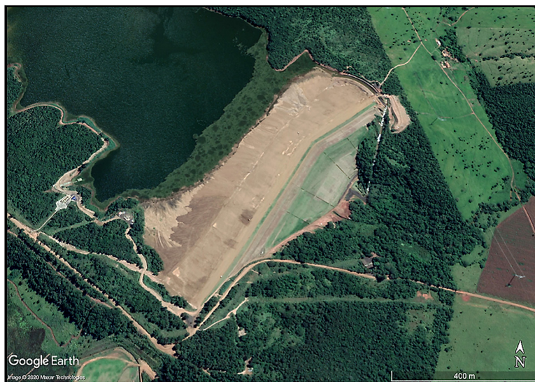
Figure 1 - Overview of tailings dam.
