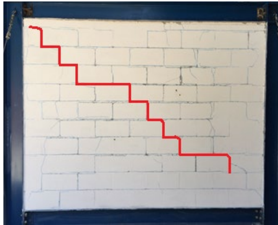
Figure 7. Typical masonry cracking after failure – PP-2-CE-0.5/2.0 (Highlighted in red: first crack register). Source: De Grandi [14]
