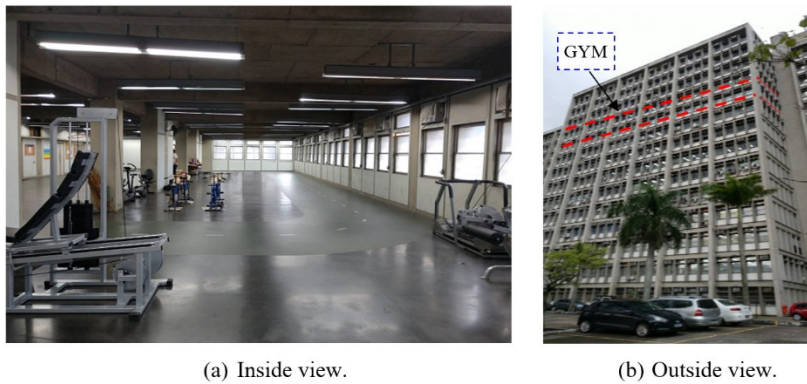
Figure 1. Investigated reinforced concrete floor.
