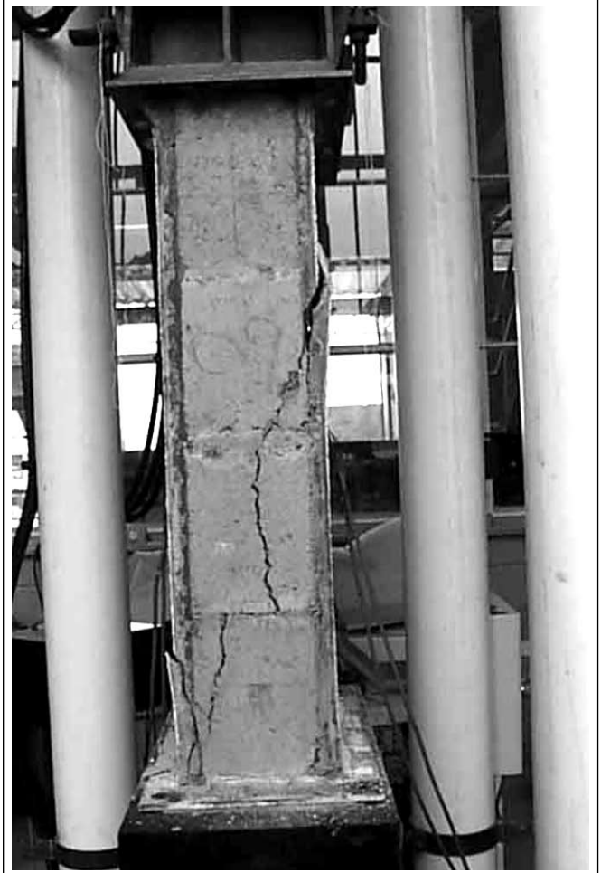
Figure 6 – Post-failure scene of P07 (steel mesh)
