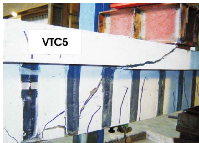
Shear crack - VTC5
