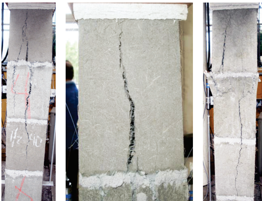
Figure 16 – Vertical cracks developed along the lateral septa
