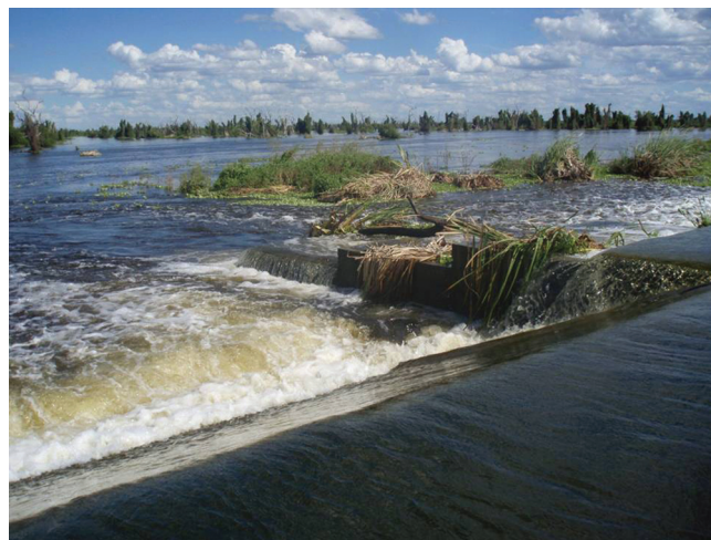
Fig. 6. View of a fish ladder (pool and weir system) operating during high flow conditions showing the contrast between discharge from spillway and attraction flow derived from the fish ladder. Note the debris inside the pools.
