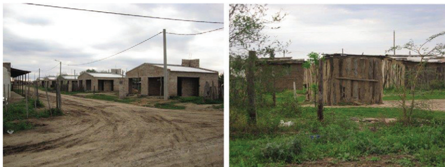
Fig. 2: peri-urban houses in Parque Industrial, Chaco, Argentina. A: built with mortared brick walls and metal roof; B: mud and grass precarious houses in the squatter settlement.
