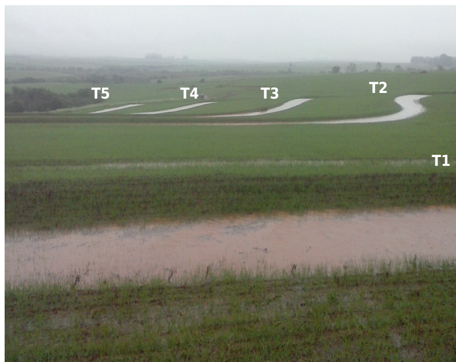
Figure 1. Terraced catchment and effect of the terraces in controlling runoff after a stormwater event (07/20/2015) with rainfall volume of 65 mm and maximum 30-min intensity of 18 mm h -1 .
