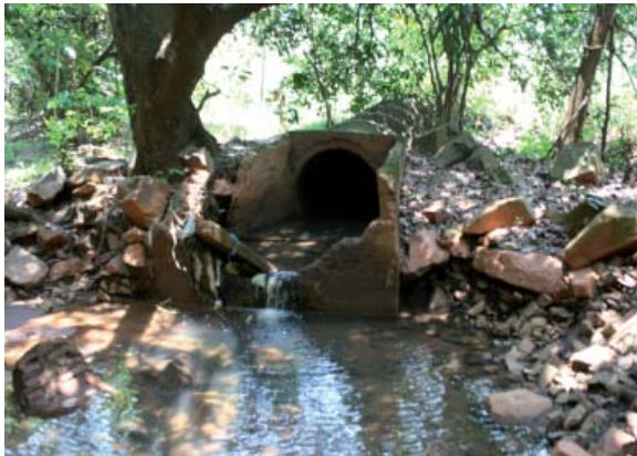
Figure 3 – Picture on November 20, 2008
