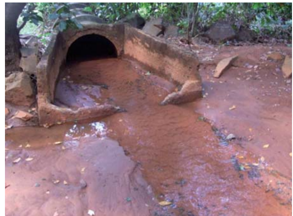
Figure 1 – Picture on November 20, 2008.
