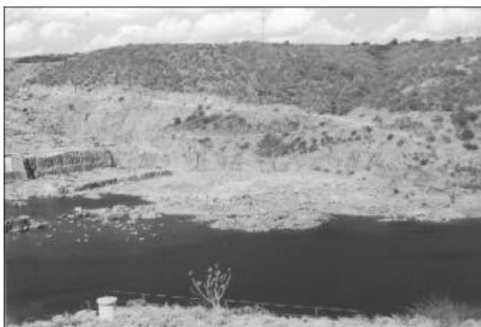
Fig. 1 — Rio São Francisco downstream from Xingó hydroelectric power dam.
