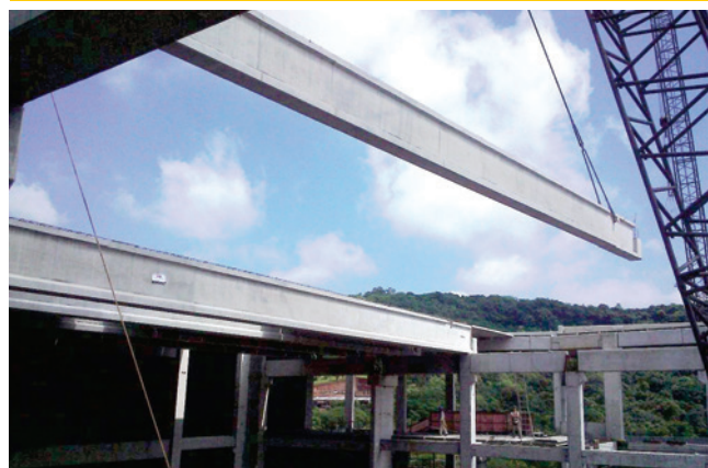
Figure 25 – Placing of the beam
