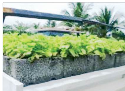
B detail of prototype with green roof with TEVA blocks on the slab
