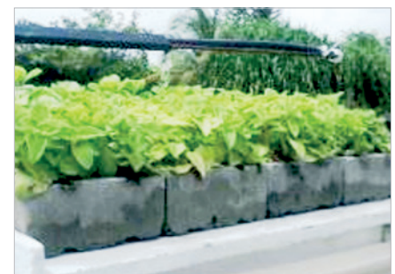
C detail of prototype with green roof with concrete blocks on the slab
