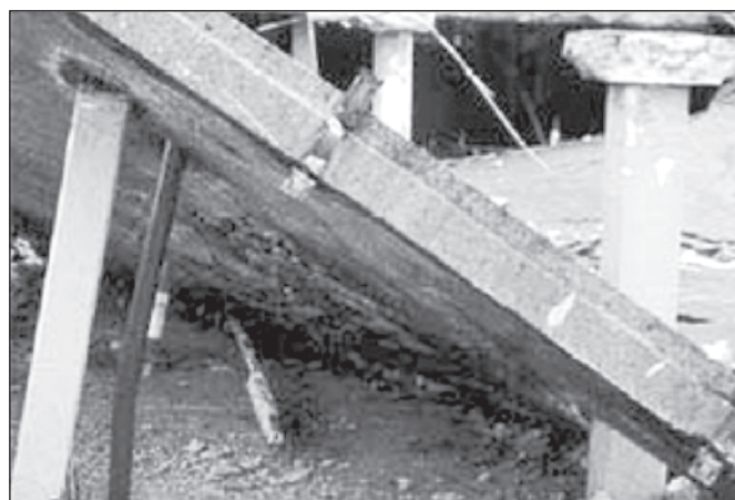
d) Piper Rows Car Park, 1997 Autor: Woods [5]
