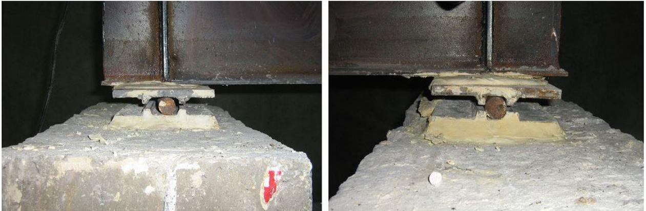
Figure 14. Composite beam support.
