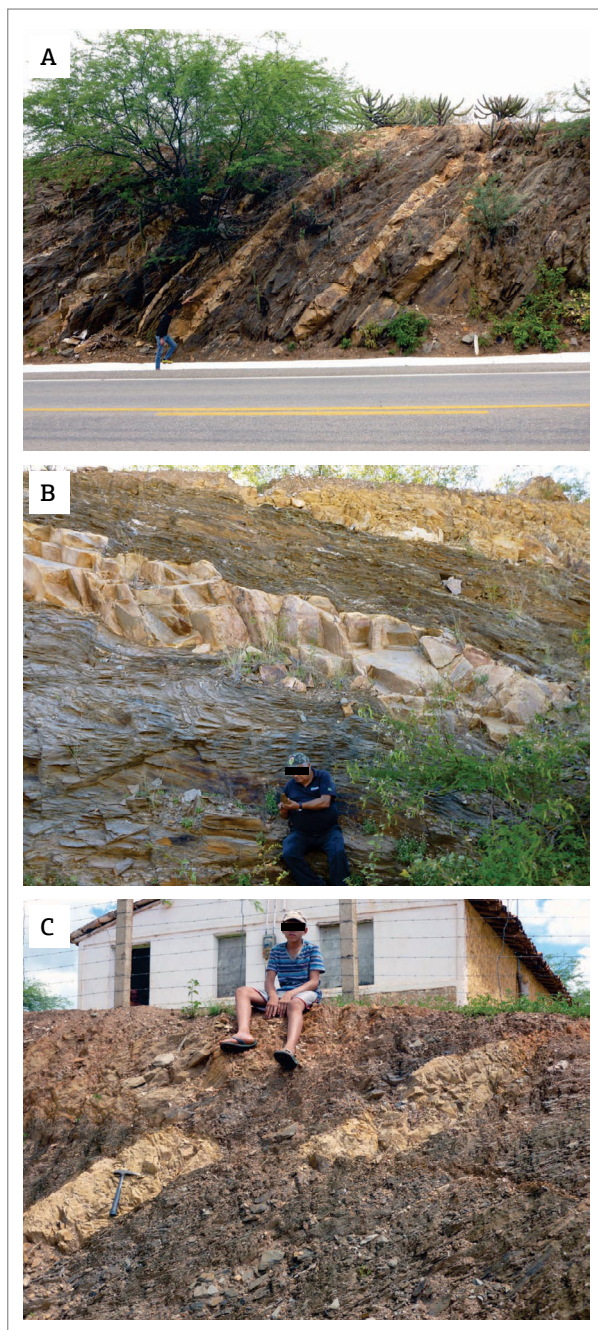
Figure 7. Photos of the felsic dykes. (A) Felsic subconcordant dykes intrusive in low-grade schists (“Salgueiro group”); km 540, BR-232, west of Salgueiro, Pernambuco; (B) felsic dykes (rhyodacitic composition) along a road cut of the “Transnordestina railway”, alternating with low-grade schists of the “Cachoeirinha Group”; north of Salgueiro, Pernambuco; (C) Stretched felsic dykes presenting “boudinage” near Curral Velho, Paraíba. Rhyolitic to rhyodacitic compositions (Brito 2014; Tab. 2).
