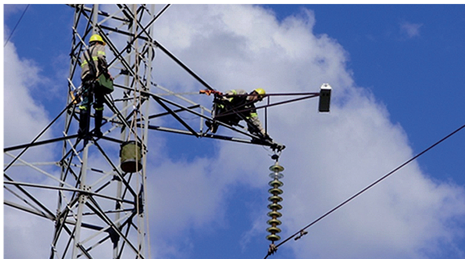
Figure 7 Installation of the accelerometer and the measurement angle digital recording system.
