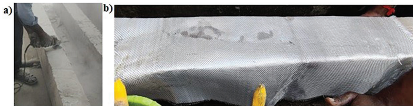
Figure 3: a) Surface treatment and b) strengthened beam process.
