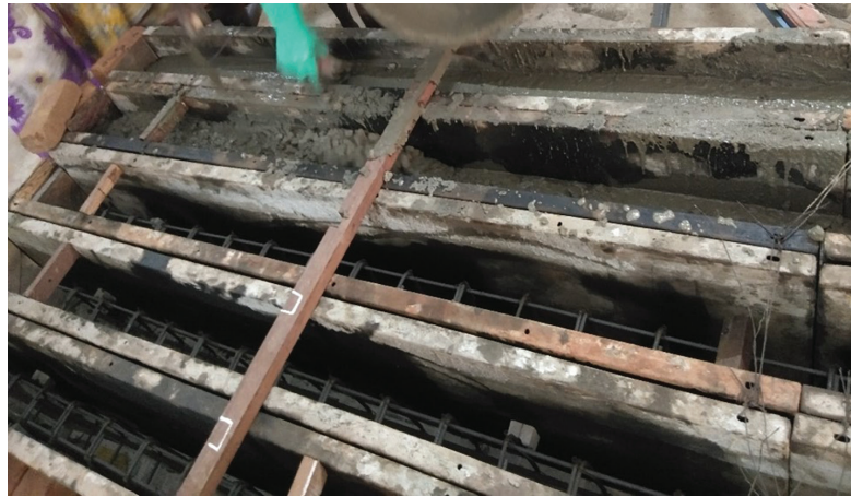
Figure 2: Casting of beam specimens.
