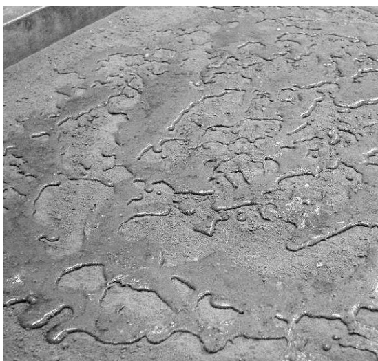
Figure 1 - Preparation of soil-cement with chemical stabilizer, noting the "impermeability" of the mixture (soil, cement and chemical stabilizer)
