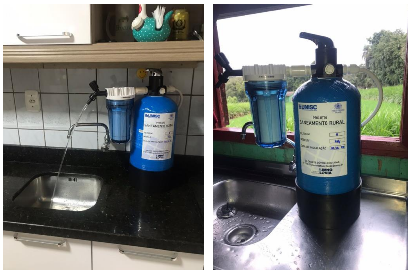
Figure 5. Filters installed at the point of use (near the kitchen sink) on two rural properties served by the project.
