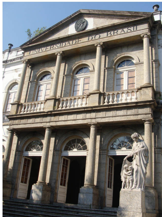
Figure. Photograph by Nardi AE. Front detail of the main entrance.
