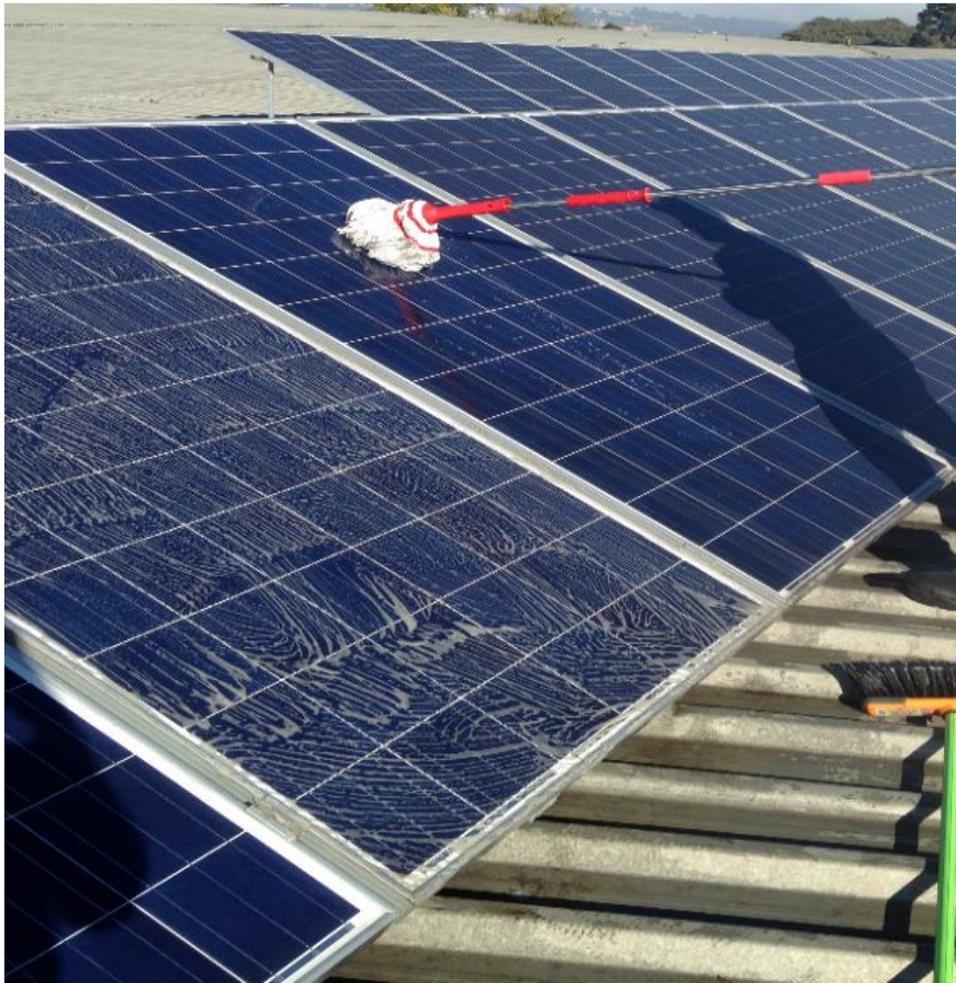
Figure 3 - Cleaning the modules in Neville
