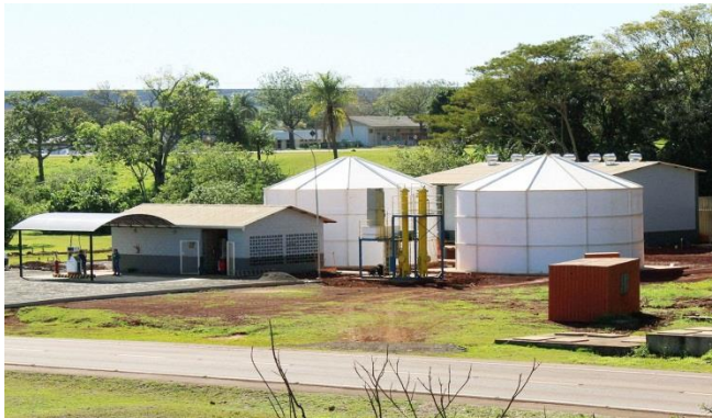
Figure 2 - Demonstration Unit (DU) of biogas/biomethane production. Installation in Itaipu Binacional.
