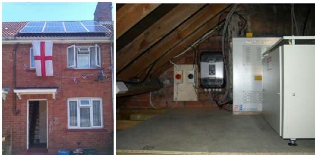
Figure 2. Photovoltaic system with storage [9] [10].
