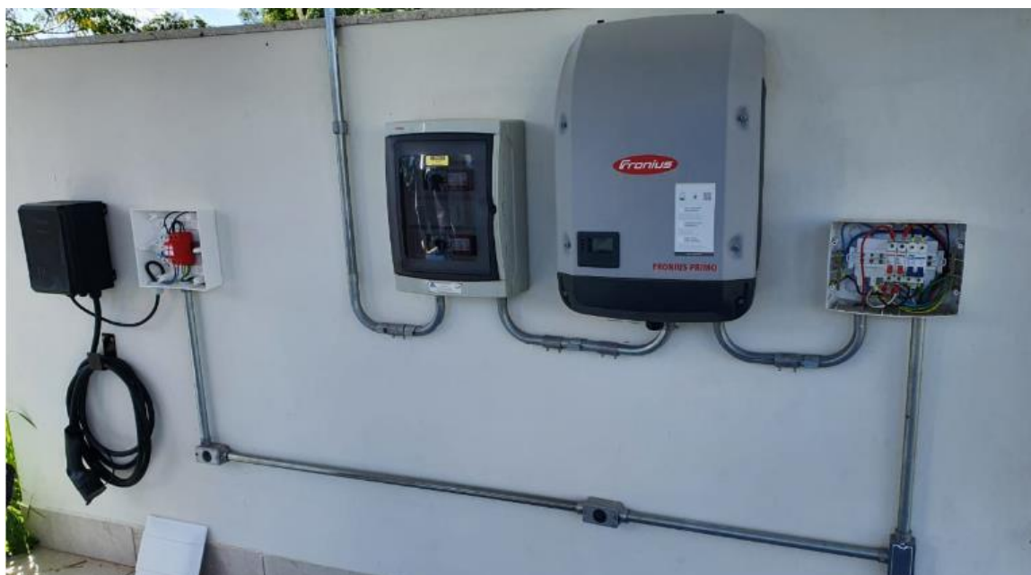
Figure 6. CARPORT wall executed to allocate the equipments
