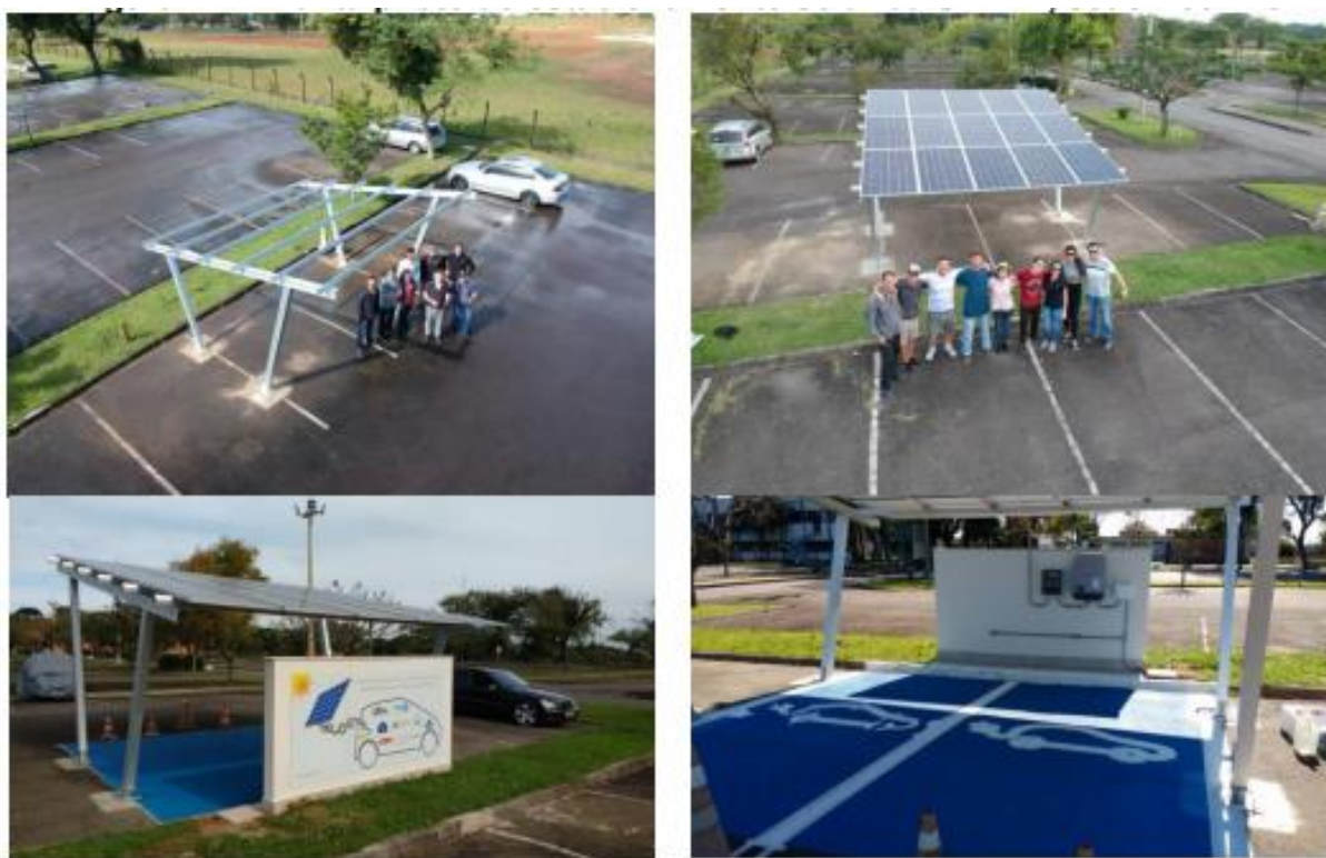
Figure 5. Pilot Project CARPORT - Result
