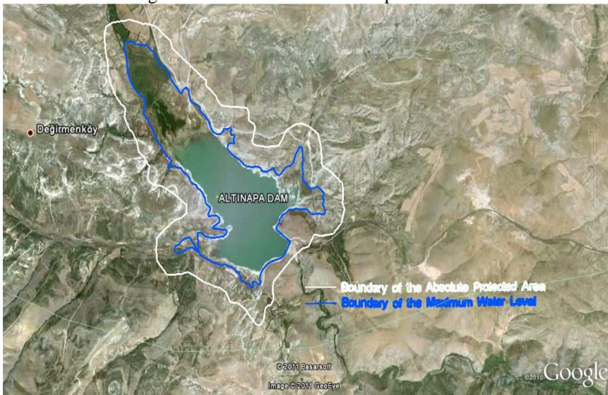
Figure 1- General View of Altınapa reservoir.
