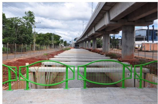
Figure 2. Luiz Rau creek after lining works. Source: Trensurb (2014).
