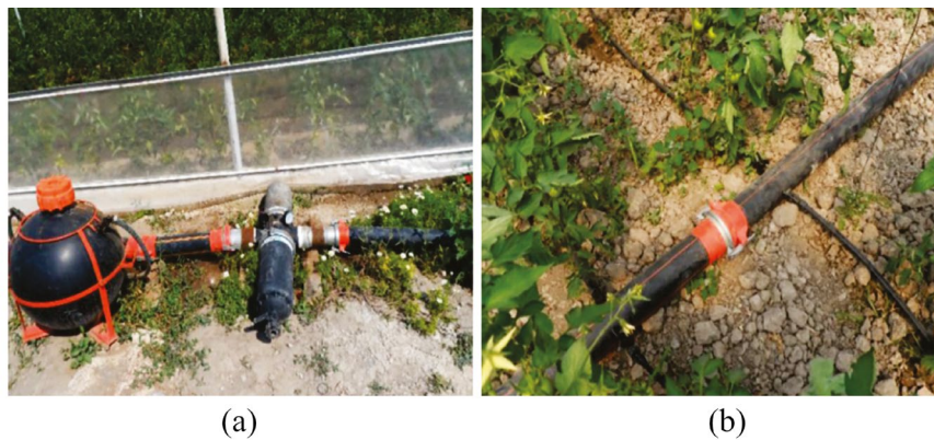
Figure 5: (a) Drip irrigation system; (b) Main and lateral pipes.
