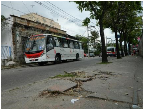
Figure 4 – Pavement conditions of bike paths/lanes in Bangu neighborhood
