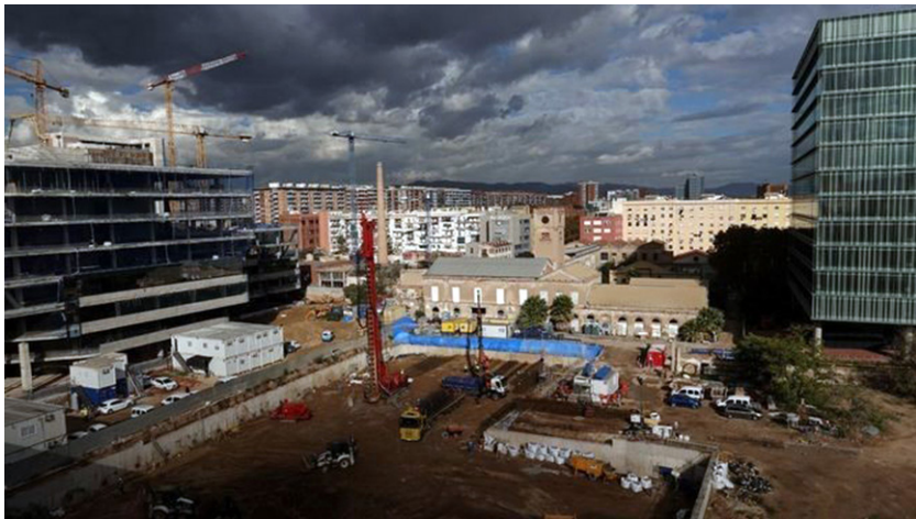
Figure 4 – Redevelopment work at Can Ricart
