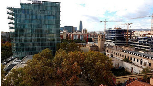
Figure 8 – The Can Ricart buildings surrounded by new constructions
