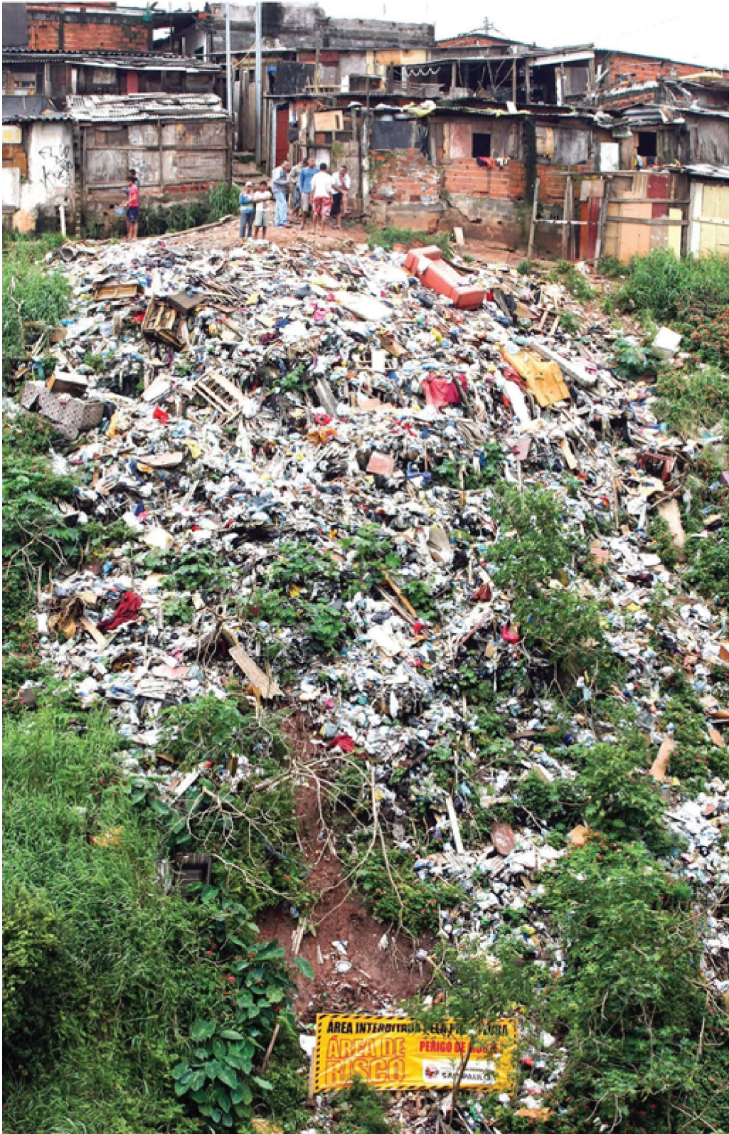
Landslide in Santa Madalena Slum ( Sapopemba neighborhood), East Zone of São Paulo.
