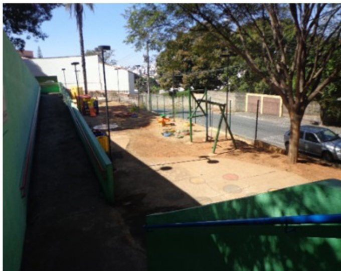
Figure 2 - View of the ECEC Tupi entrance and playground
