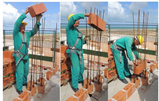
Figure 13. Block laying.
