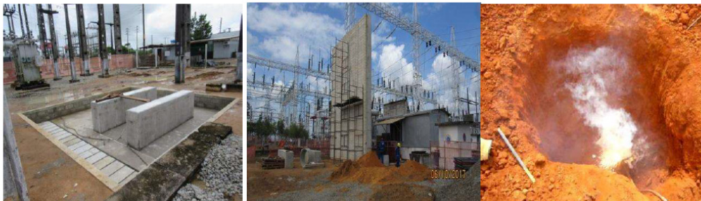
Figure 4. The construction activities.
