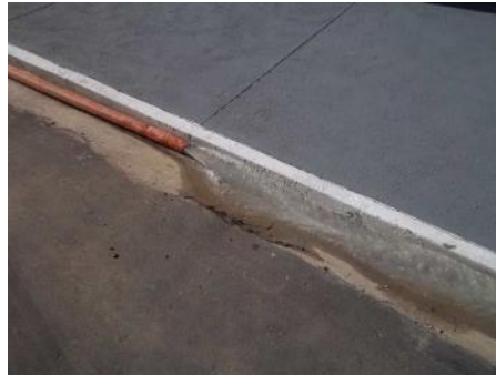
Figure 3. Dumping water in urban drainage network. Source: the authors.
