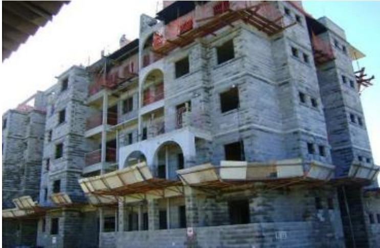
Figure 9. Construction tower view. Source: the authors.
