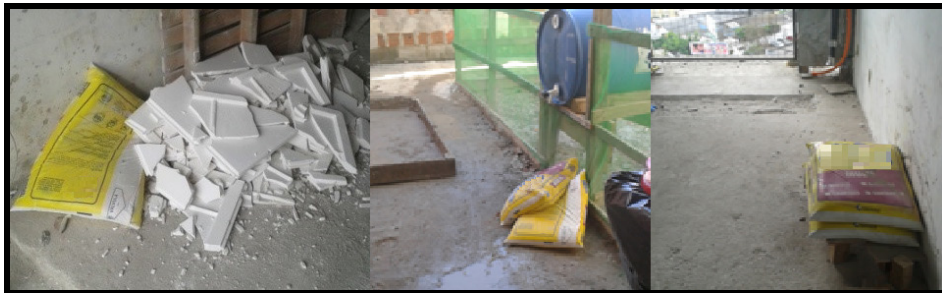
Figure 20. Deviations in the transport of mortar bags. Source: Authors.
