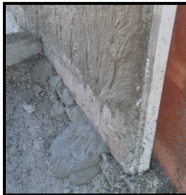
Figure 19. Application of mortar with low consistency in construction work 7. Source: Authors.
