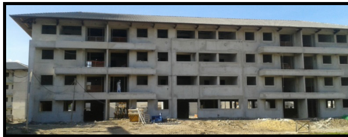
Figure 16. Facade in the construction work 7. Source: Authors.
