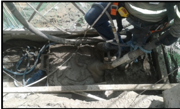
Figure 17. Mortar return containment in construction work 5. Source: Authors.
