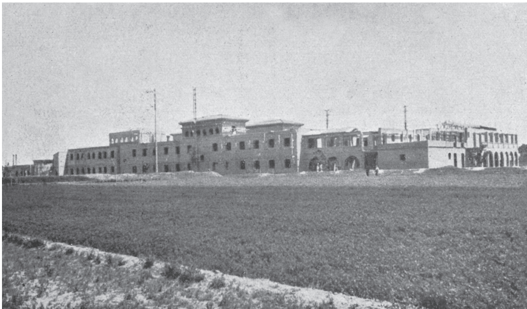
Figure 3: Construction on the El Cid Municipal Hospital Municipal for Infectious Patients, c.1943 (Vidal Jordana, 1946, p.48)
