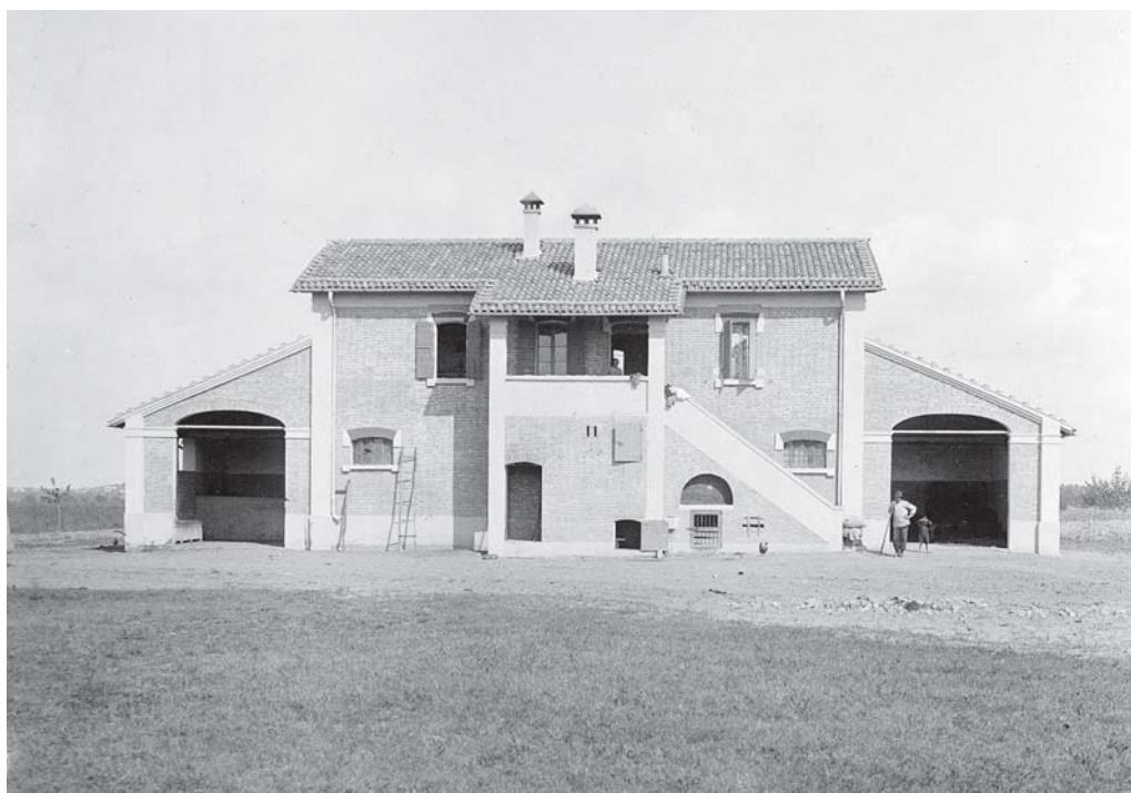
Figure 16: A standard-type farm such as were mass- constructed in bonified areas, here in Agro Romano. Note the clear-cut separation between spaces devoted to human housing (top floors) and spaces devoted to animals. Also note the absence of visible 'domestic' water (Archives..., 1925)
