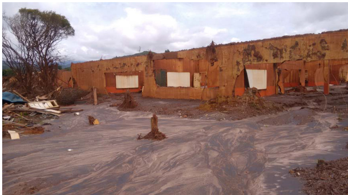
View of the remains of a public school completely destroyed by the Fe ore waste (Photo: Rodrigo Aguiar).
