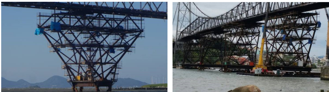
Figure 23: Auxiliary structure tower assembly.
