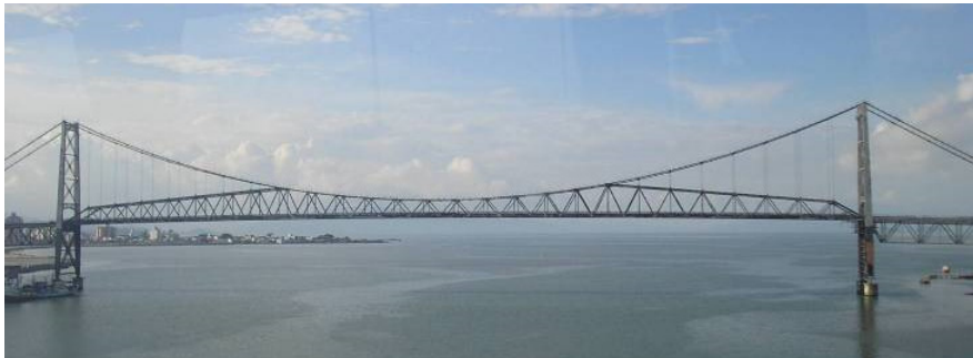
Figure 2: Main span of the Hercílio Luz Bridge (339.5 meters long).
