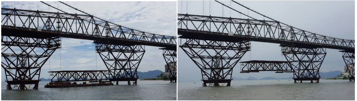
Figure 24: Transportation and hoisting of an auxiliary structure truss part.
