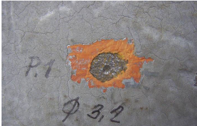
Figure 11: Hardness test in main structural elements.
