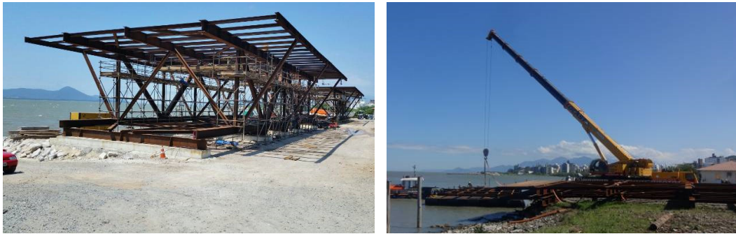
Figure 22: (a) Structure pre-assembly on site (b) Structure transportation by floating devices.
