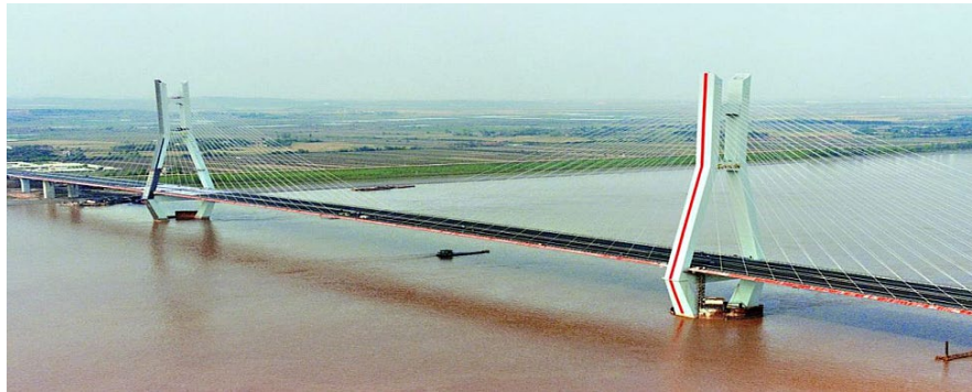
Figure 1: Wuhan Junshan Yangtze River Bridge.
