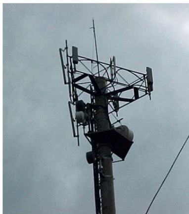
(a) Photographs of the tower
