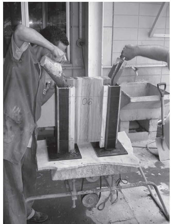
Figure 4. Concrete being poured in specimen.
